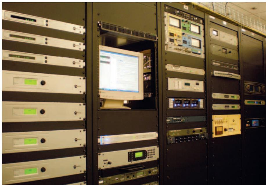
**KUNV's rack space in the TOC includes Omnia 6EXi and Omnia One processors, Axia engines and audio nodes, Comrex Access, Arbitron PPM encoders, Public Radio Satellite System hardware, streaming server/encoders and iMediatouch skimmer. Also at work is gear from Sage, Broadcast Tools, DaySequerra, QEI, Orban, Moseley and Belar, among others.**
