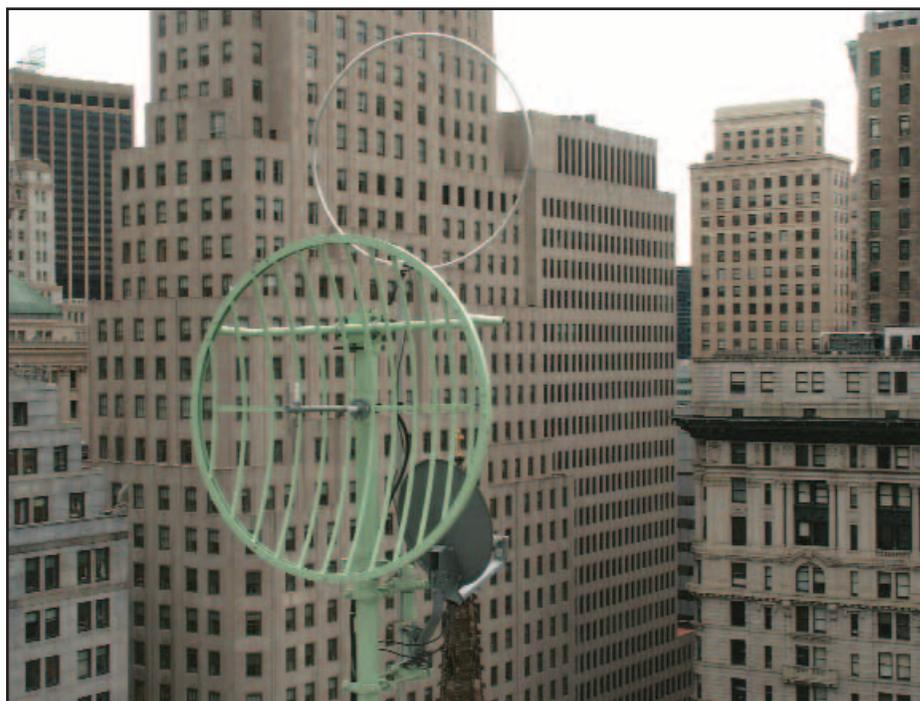
*Fig. 7: The STL antenna, AM loop and DirecTV antenna mounted on the roof. The Mark grid dish is painted the same color as the building penthouse.*
