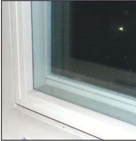
*Fig. 4: This inside plate glass window reduced outside noise by over 60 dB.*
