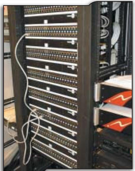
*WCBS in New York has installed a Radio Systems StudioHub system, which includes an RJ-45 patch panel for manual switching. Each RJ-45 connector carries a balanced, bidirectional stereo pair. Gray switches in the center row of each rack control normalizing between the upper and lower rows.*
