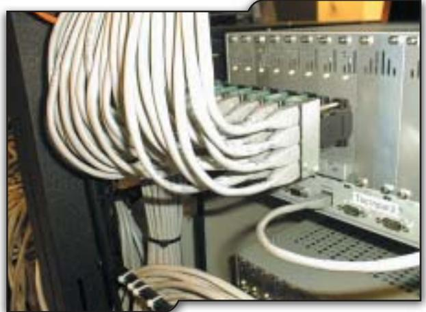
*A close-up of the Radio Systems StudioHub rear panel shows how the multiple RJ-45 connectors are interfaced to the rack frame.*
