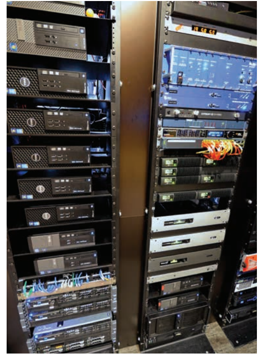
Left rack: Op-x automation and VoxPro PCs; right rack: codecs and AoIP studio engines
