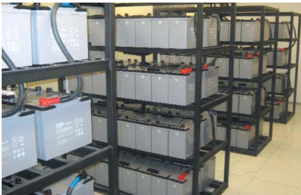
**UPS on steroids:** RFE/RL's basement holds enough backup charge and emergency cooling to keep the most important systems operational during even lengthy outages.
