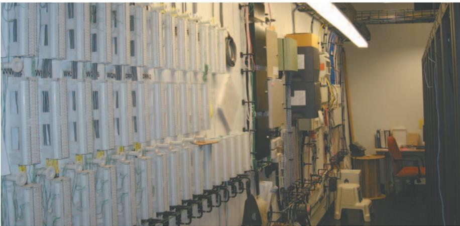
Tech Center Backboard. GPIO cross-connects for satellite receivers are in foreground.
